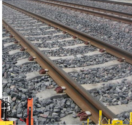
Track panel laying
